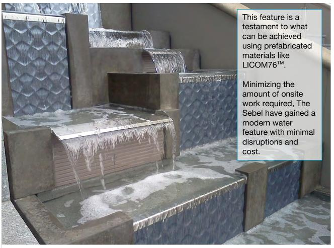
The water feature was designed in 3 parts after extensive onsite measurements. The first water wall (1535mm x 755mm) is clad to the existing wall and delivers water from a trough above through a custom designed spillway.
